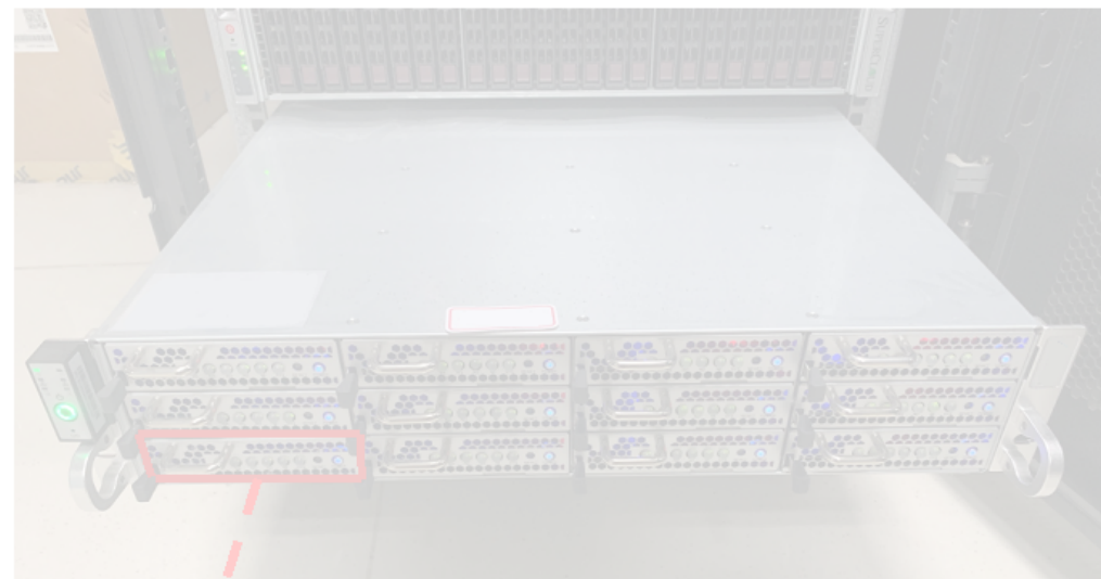
(b) The overview of a physical server.
