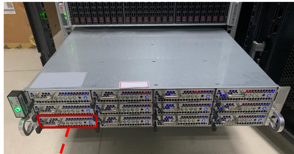
(b) The overview of a physical server.
